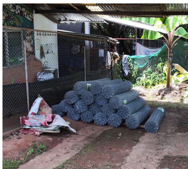
Everything ready for the new fencing
